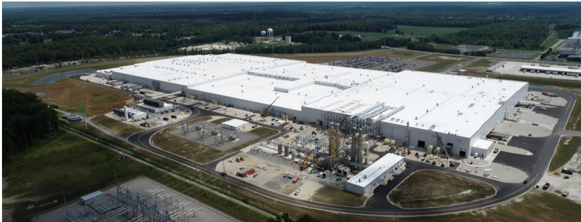
Figure 2: The Exterior of the Ultium Cells Facility in Warren, Ohio
